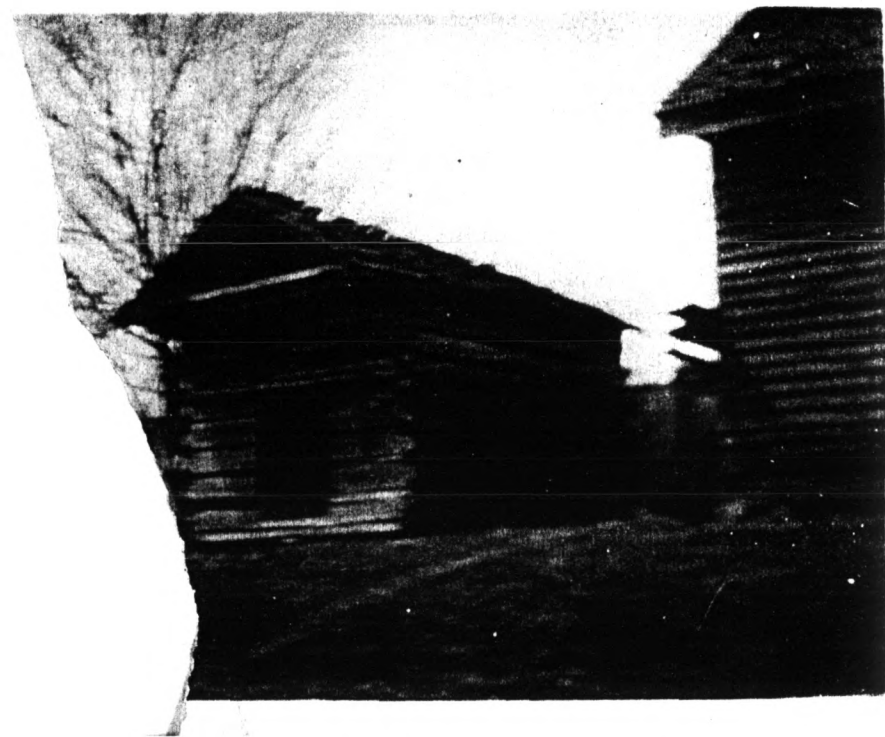
Buildings behind Keener-Johnson House ca. 1915. Building on right no longer extant
